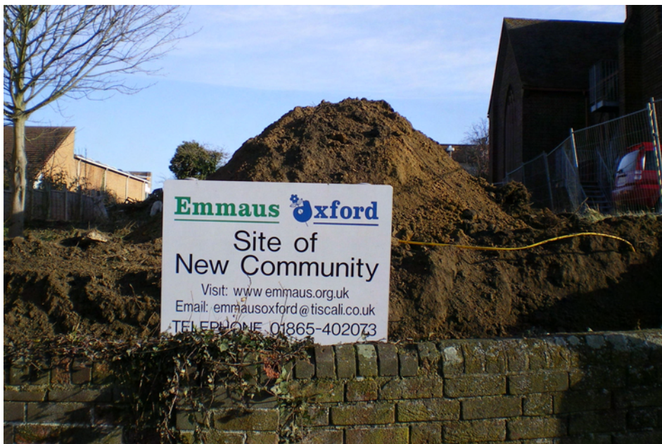
Above: Work has now started on site at Emmaus Oxford
