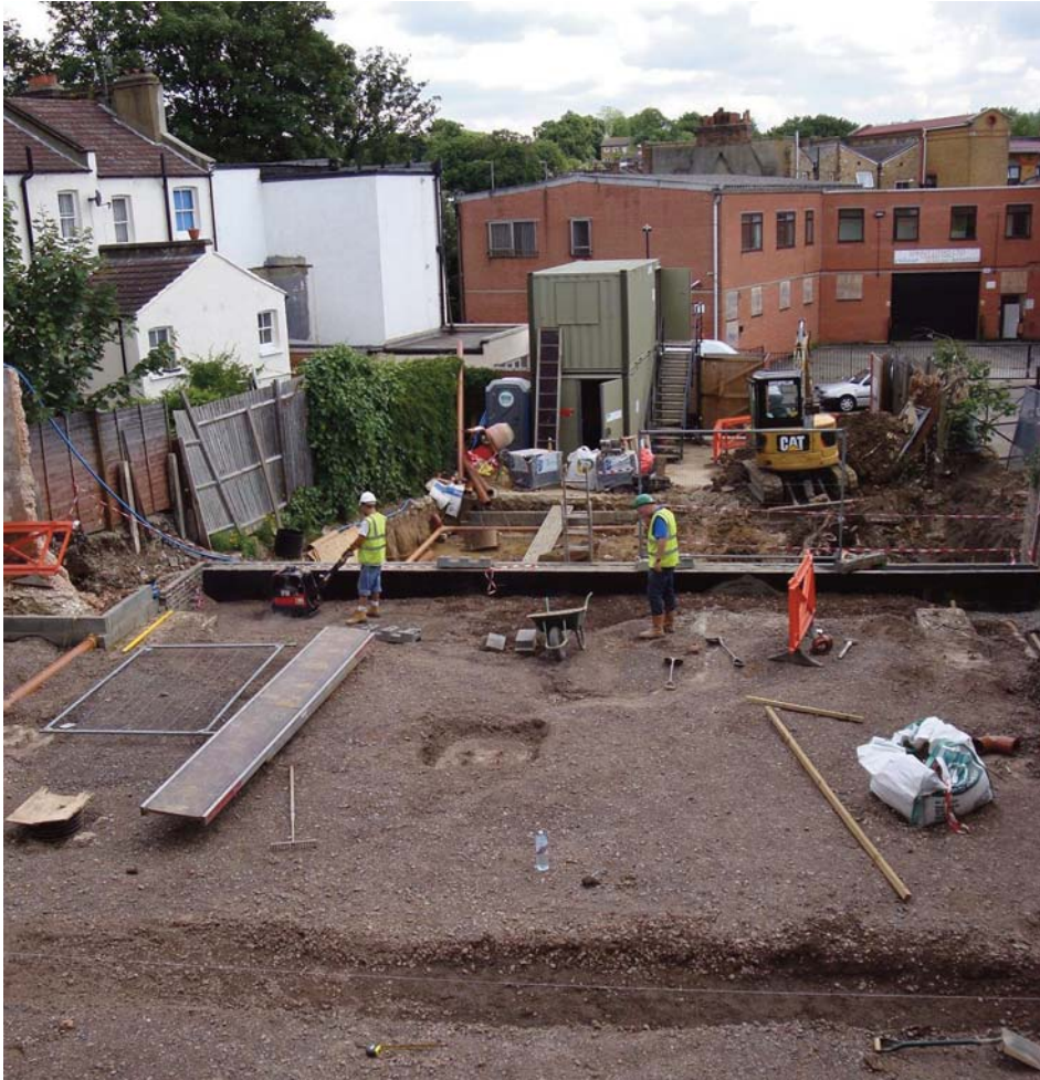
Above: Work in progress
